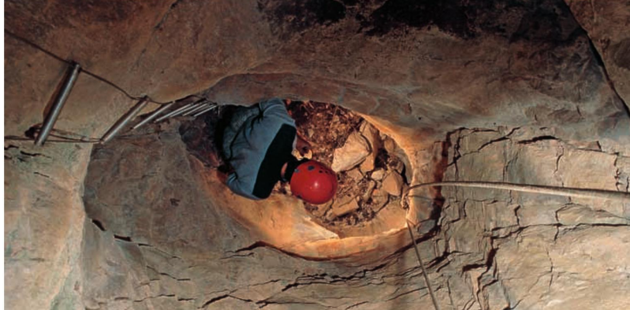
Vertical excavation by fire setting 8 m deep, la Pinée, L'Argentière-la-Bessée (France) © Inrap
